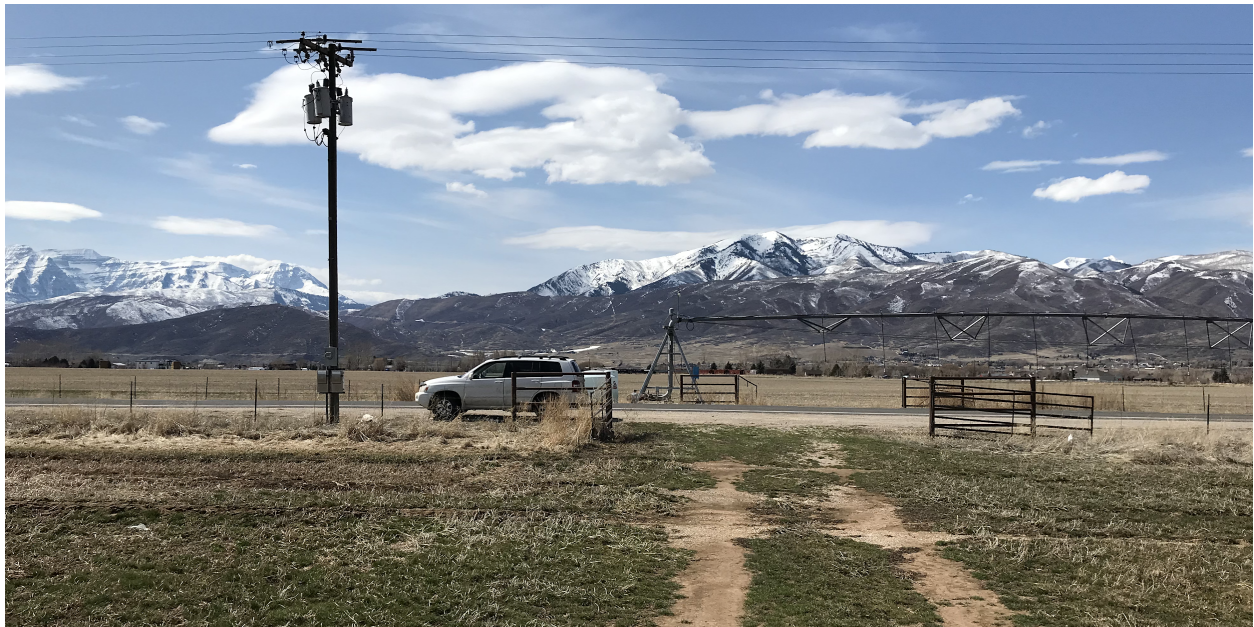
View from pivot irrigation field looking west at the North pivot power drop across S 1200 W St (South field Rd) to a half-circle pivot on the west side of the road.
