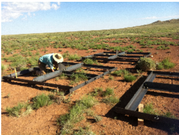
Building the anchor baskets for RIM
