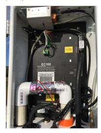
Around 11:25 EDT I rserial'd to the EC150 on S15 (port 5). The pressure setting can be changed with the "O" command. It is a hassle because we don't know how to disable the unprompted output, and so the menu prompts are interspersed in the binary output.
