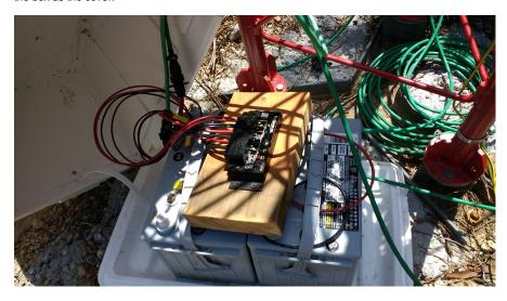
Tying off or looping the cables at the top with the controller will ensure they will always be well above the waterline for any that gets into the box. At this time towers tse05 and tse07 have been flipped.
